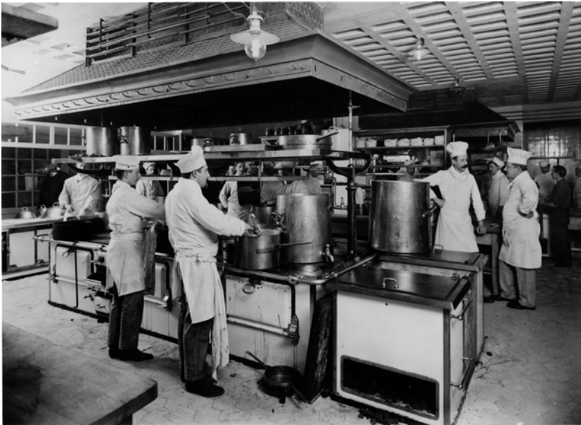
FIGURE 1.12 Cooks in the main kitchen of the Esplanade, one of the first cellar kitchens in a Berlin hotel to feature mechanical ventilation, ca. 1915 Image credit: Landesarchiv Berlin
